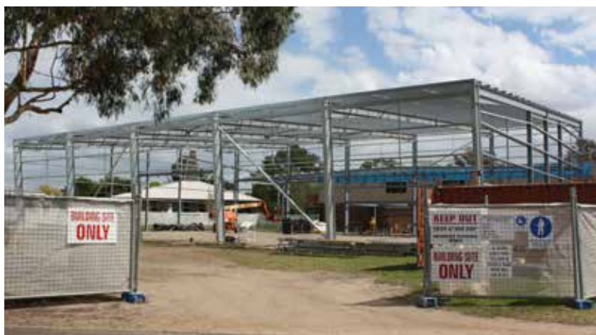
Photo: Work in progress at Garnsey Campus.
